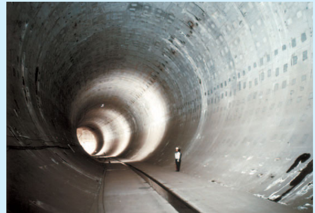
Inside a storm water reservoir. When full, the system can hold 540,000 tons of floodwater.
