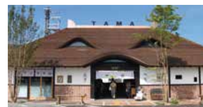
猫の顔と日本の伝統工法檜皮葺(ひわだぶき)屋根の貴志駅 DESIGNED BY EIJI MITOOKA + DON DESIGN ASSOCIATES
