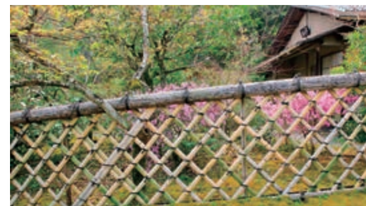
▲ This bamboo fence is at Koetsu Temple in Kyoto, which is famous for its Japanese garden. Split bamboo is tied in a rough diamond pattern, thus distinctively providing a view of the other side of the fence.
