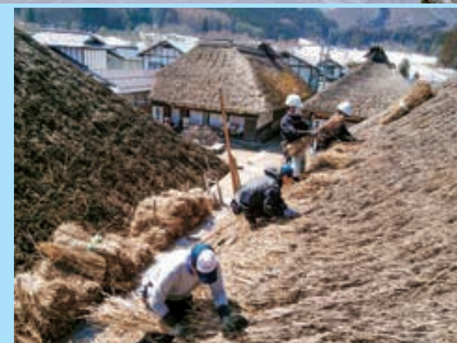
With craftsmen called kayate taking the lead, all residents cooperate in rethatching the roofs.
